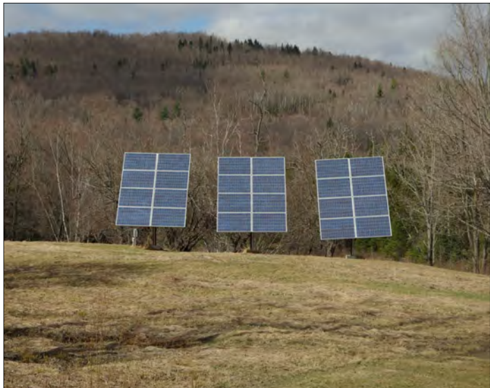
Some Landgrove residents already have deployed renewable energy systems such as these solar-tracking photovoltaic panels.
