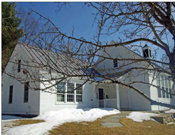
The recently expanded town hall is an important public building.
